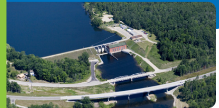
Five Channels Dam
